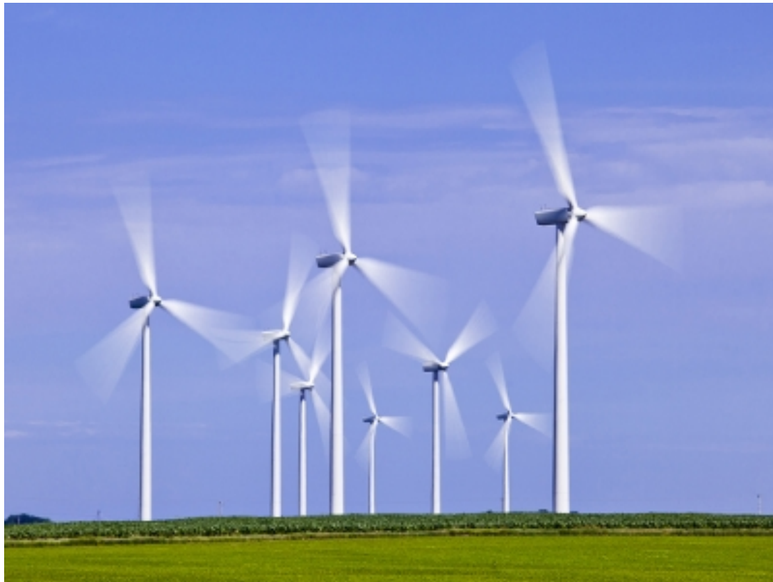
The Streator Cayuga Ridge South Wind Farm has 300 MW capacity of electricity. | Photo courtesy of Greater Livingston County Economic Development Council
