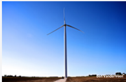
The Gratiot County Wind Project, the largest wind installation in Michigan, operates more than 100 turbines.
